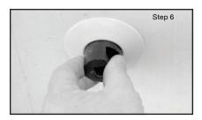
Step 6. With the escutcheon in place and with pipe-thread sealant applied to the pipe threads, hand-tighten the sprinkler into the sprinkler fitting using the TYCO W-Type 25 Installation Wrench with the wrench prongs fully engaged with the sprinkler wrenching notches. The wrench prongs are designed to engage the wrenching notches in the sprinkler body, and are also uniquely spaced to align with the sprinkler wrenching notches in one position.
