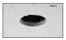
**Step 5.** Ensure that the ceiling/wall is smooth for the escutcheon to sit against and that the distance from the ceiling/wall surface to the sprinkler fitting is appropriate. As shown in Figures 5 and 6, the take-out dimensions are 1 inch for pendent sprinklers and 1-5/16 inches for horizontal sidewall sprinklers.
