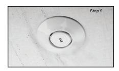
**Step 9.** After installation is complete, ensure that the RAVEN Escutcheon is held fast against the mounting surface and sits squarely against the ceiling around its entire perimeter.
