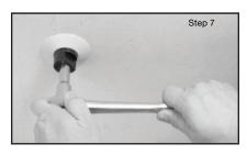
**Step 7.** Wrench-tighten the sprinkler using only the TYCO W-Type 25 Installation Wrench (Ref. Figure 3).
