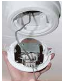
Step 2: Terminate Cable
