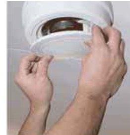
Step 3: Fit Speaker to Housing
