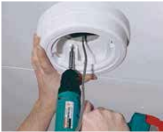
Step 1: Secure Housing to Mounting Surface
